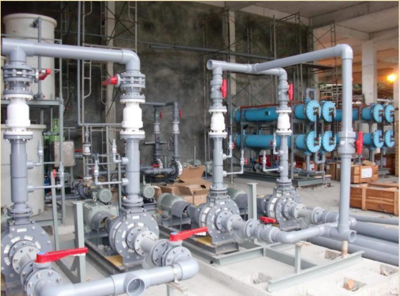
SYSTEM ON INDIVIDUAL SKIDS, assembled at site 2x72 KGS/HR, SEM CALACA, Philippines
