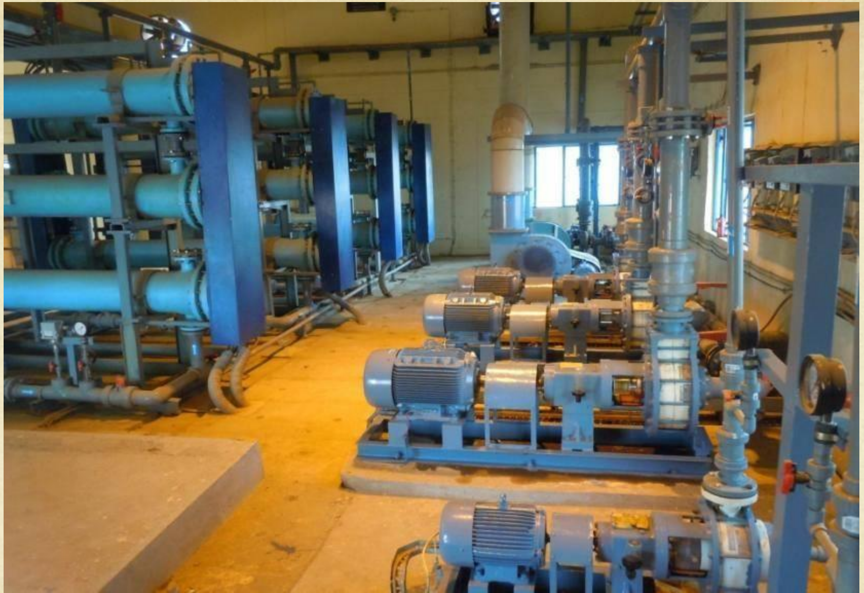
4 x 50 KGS/HR SEA WATER ELECTROCHLORINATION SYSTEM CW CHLORINATION , LANCO UDIPI POWER PLANT
