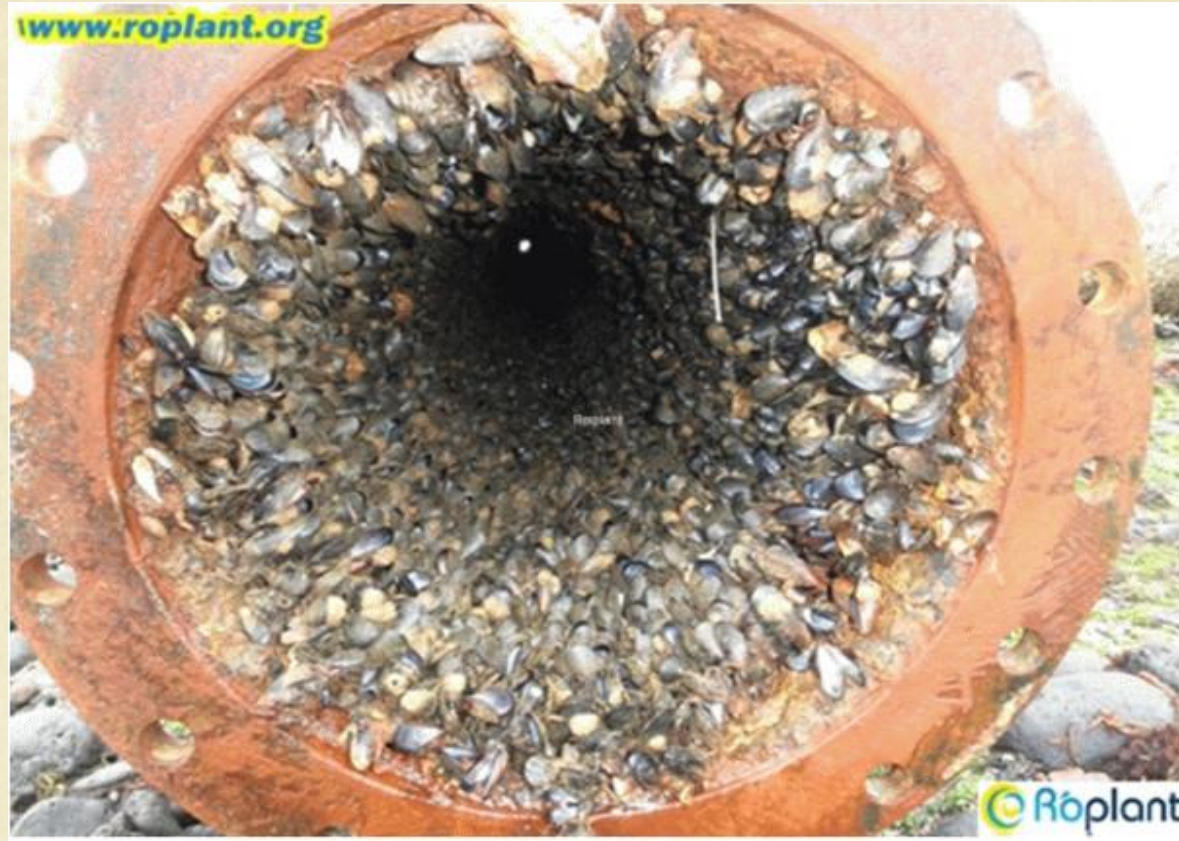
Shells and Bio Fouling inside Sea Water Pipe
