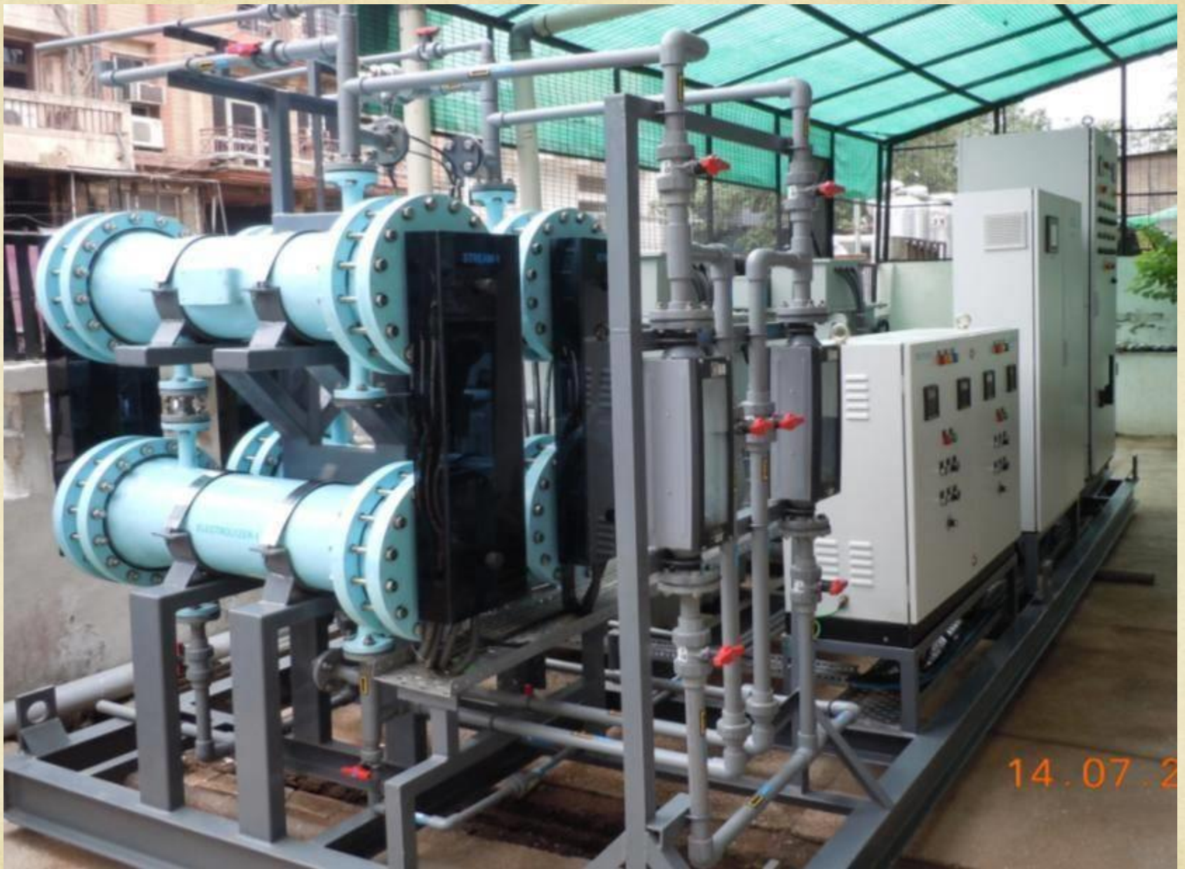
COMPLETE SKID MOUNTED BRINE BASED SYSTEM 2 x 5 kgs./hr. for JSW Bellary.
